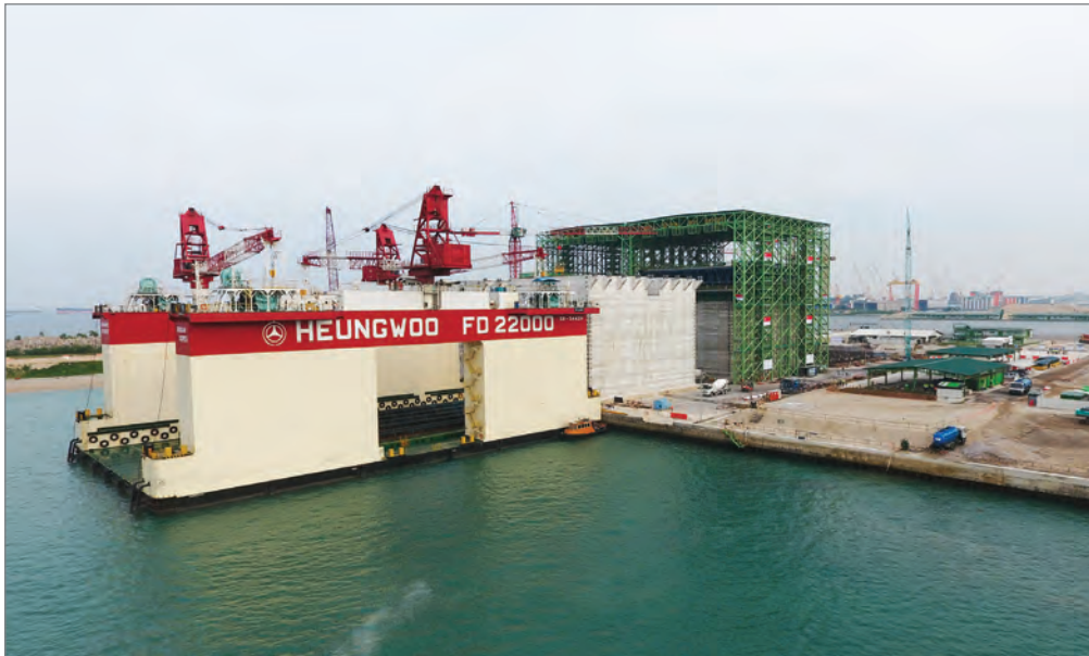
싱가포르 - Tuas terminal phase 1 reclamation wharf construction and dredging (2016.03 ~ 2019.04)
